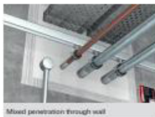
Mixed penetration through wall
